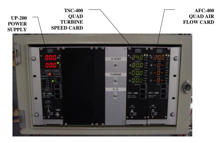
The EFC 4x4 Card cage is a pre-wired system that supports the PS-100, UP-100, UP-200, UP-500, TSC-400, FRC-400, AFC-400 products from EFC. The card cage and back plane can be designed to handle the following configurations:
